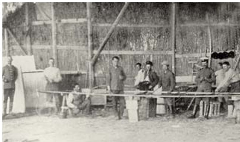
Assen Jordanoff, seventh from left to right, during repair works on Abatross' wing. Mustapha Pasha airfield.
